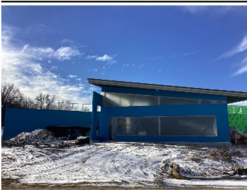
Phase 2A Community Center: Northwest side of the building (Looking South)
