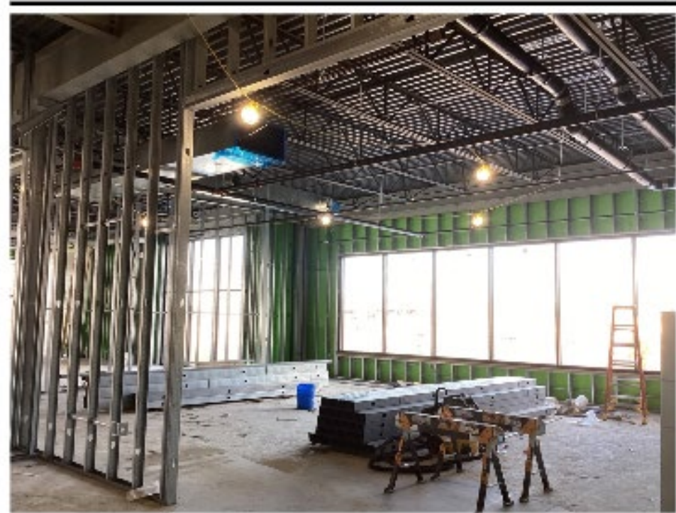
Phase 2A Community Center: Aerobics (Looking NW)
